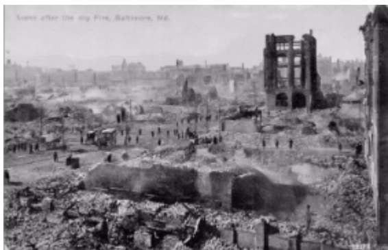
Figure 1.1 Aftermath of the 1904 Great Baltimore Fire (source: Wikipedia)
